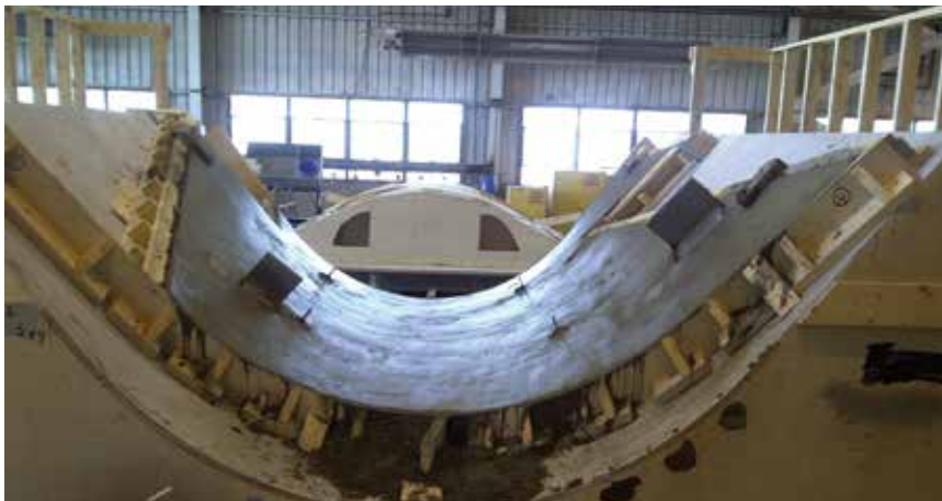
The precaster had to cast a variety of curved panels with many different radiuses, many of them tight. These curves required the back of the panels to be formed up so the concrete stayed inside the form at the panel was cast.
